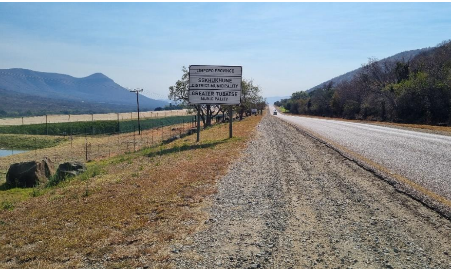
Paved Road to Site
