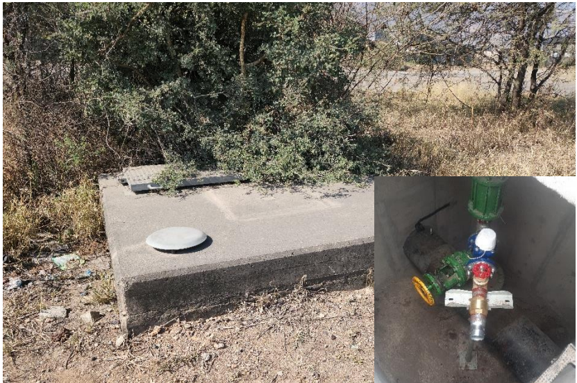
Water Source at Entrance
