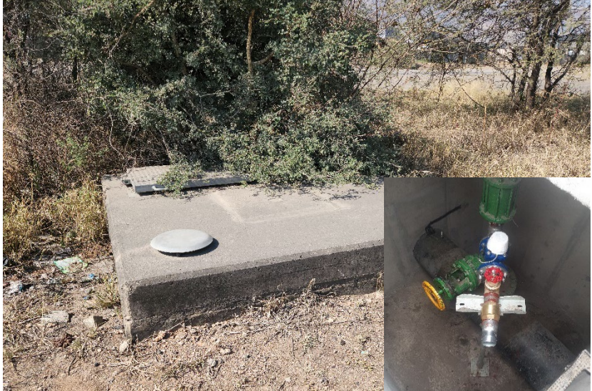
Water Source at Entrance
