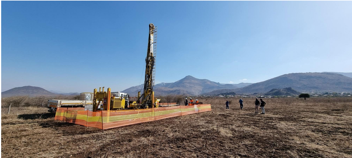
Figure 1: Atlas Copco CS-1500 drilling drillhole E019
