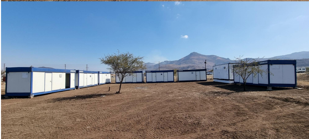
Figure 4a/4b: Geological office and drillers lay down area
